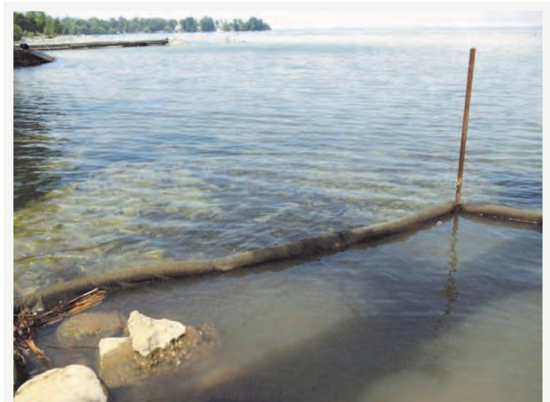
Turbidity curtain must ensure sediment does not leave work area.
